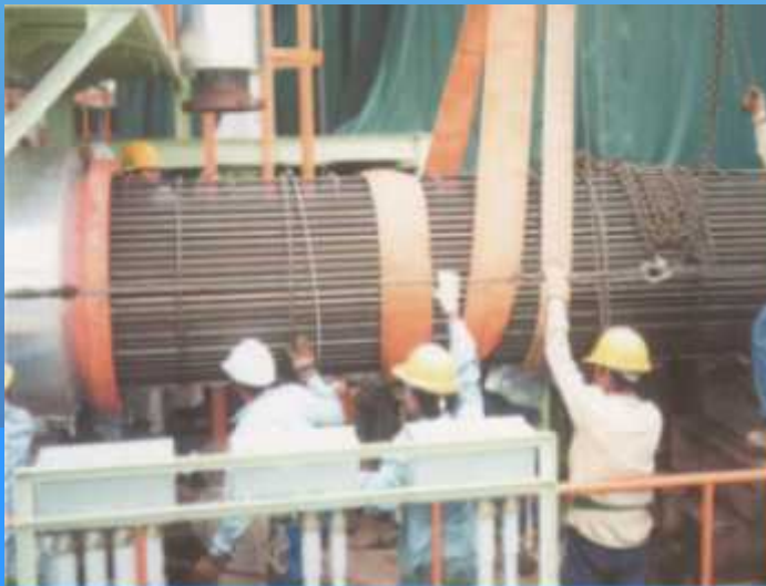
Cleaning & Repair for Heat Exchanger Tube-Bundles
