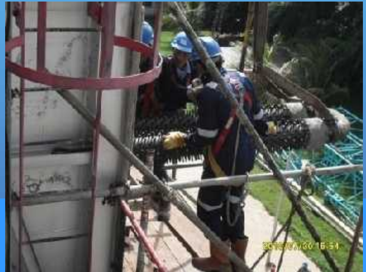
Re-tubing for Radiant Tubes
