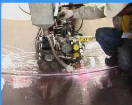
Welding Shell Kiln
