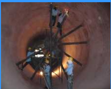
Welding Shell Kiln
