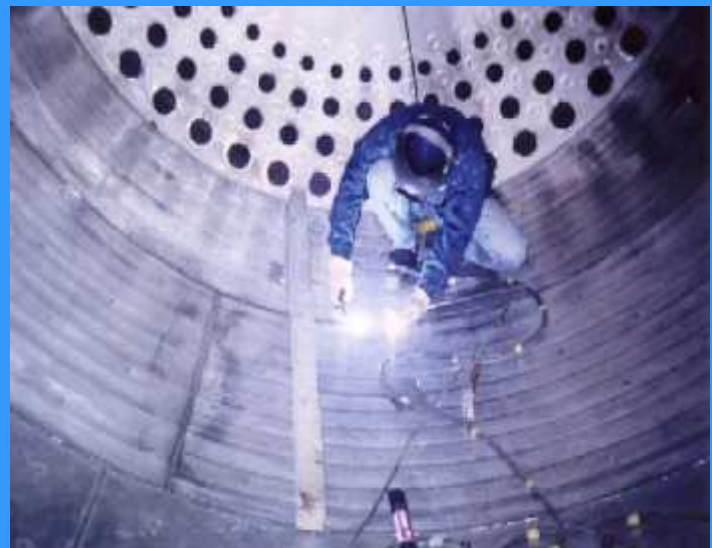
Repair for Shell of Dryer
