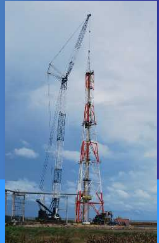
Installation Derrick Stack & Flare Tip
