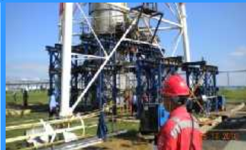
Replacement for Flare Shell Gas Drum
