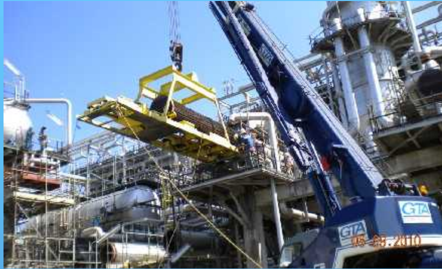
Cleaning & Repair for Heat Exchanger Tube-Bundles
