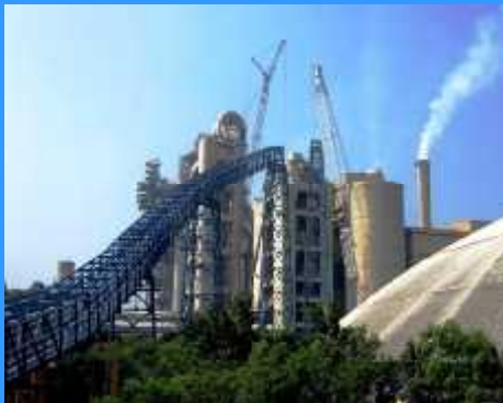
Installation for Conveyor
