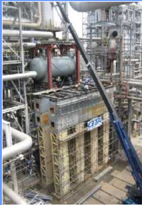
Installation of Steam Drum for Revamping Work
