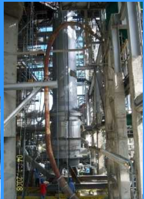
Replacement for Catalyst Cooler
