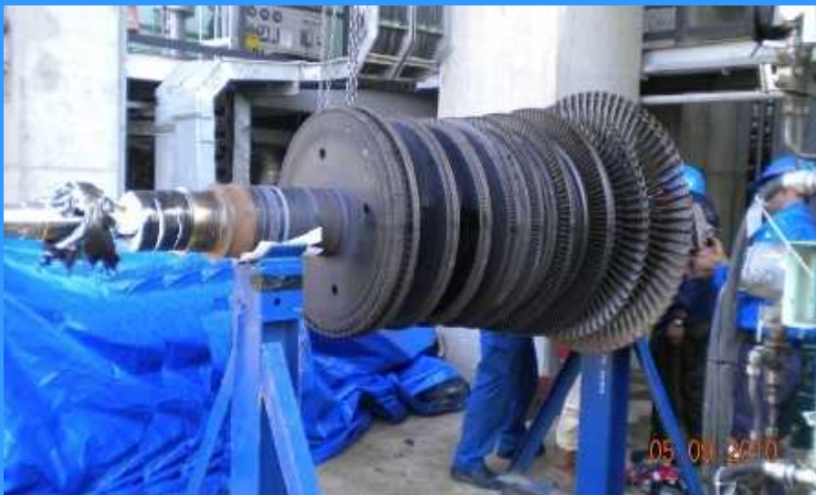
Over Haul for Turbine Compressor
