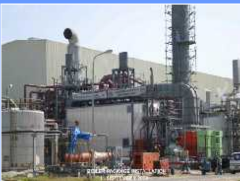
Installation for Boiler Package
