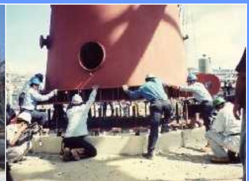
Installation for Reactor
