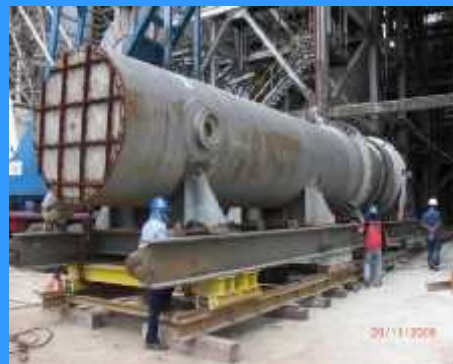
Replacement for Catalyst Cooler
