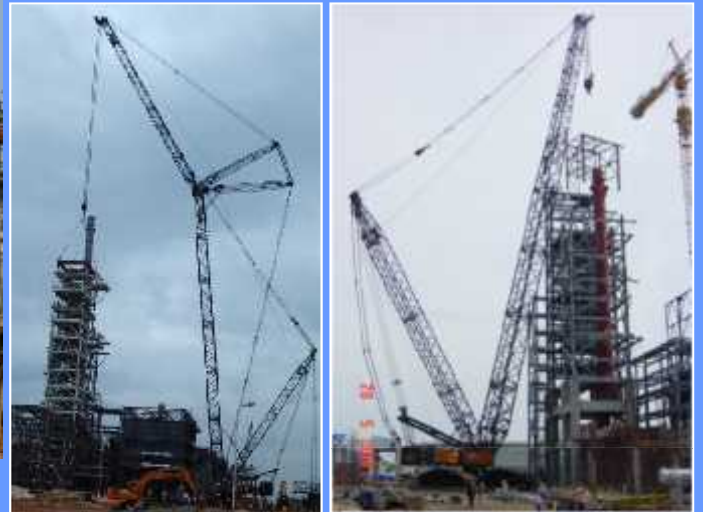
Assembling and Installation for Steel Structure by Module Method
