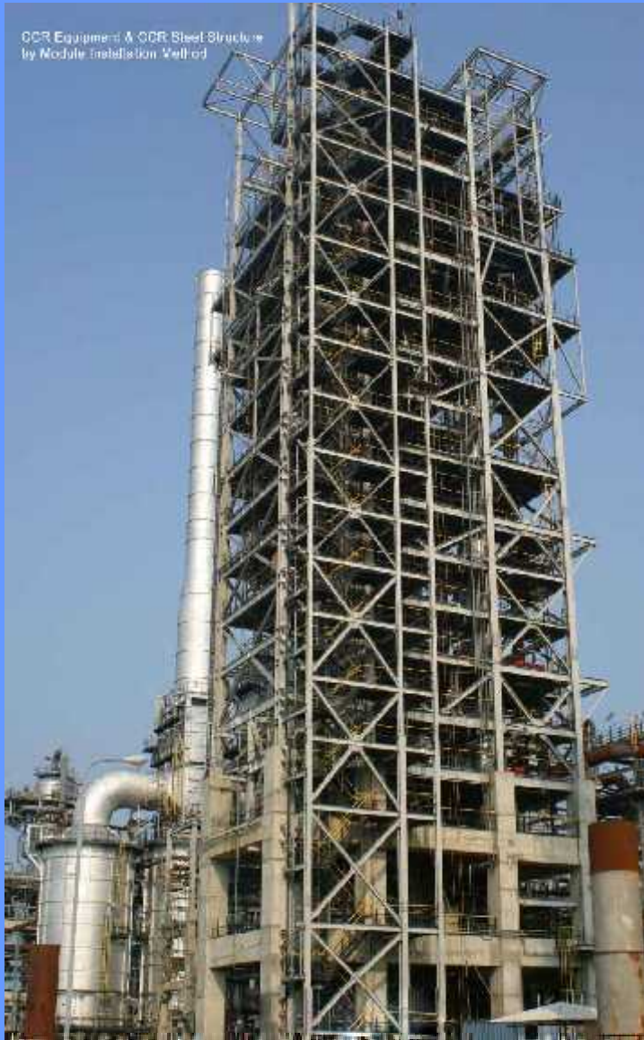
Assembling and Installation for Steel Structure by Module Method
