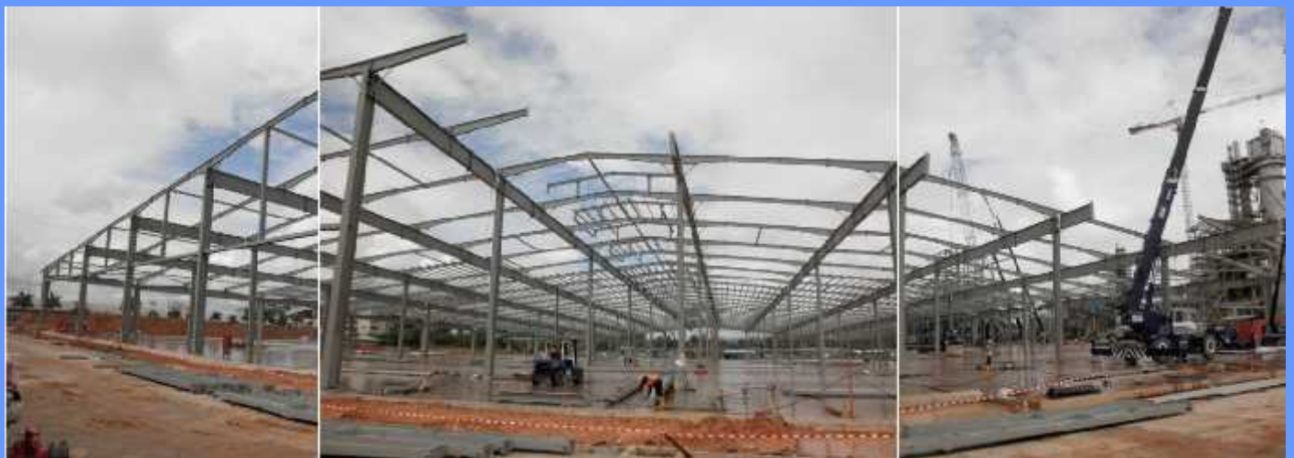
Assembling and Installation for Building Steel Structure
