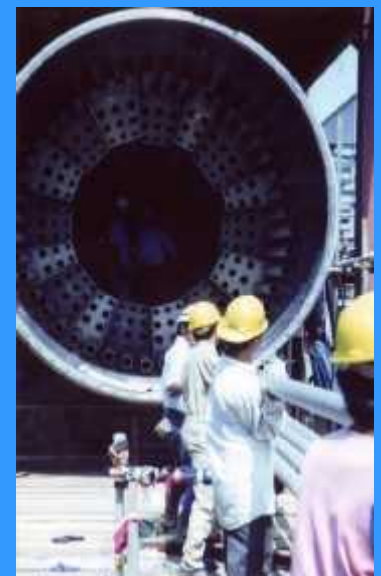
Re-tubing for Dryer's Tubes
