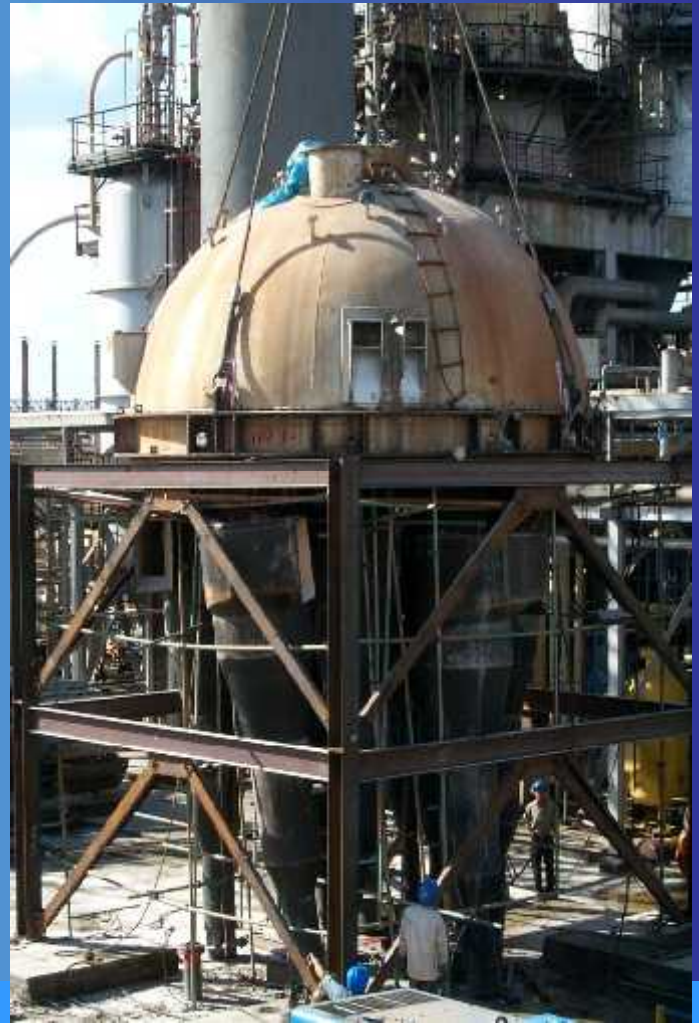
Repair for Planum of Regenerator
