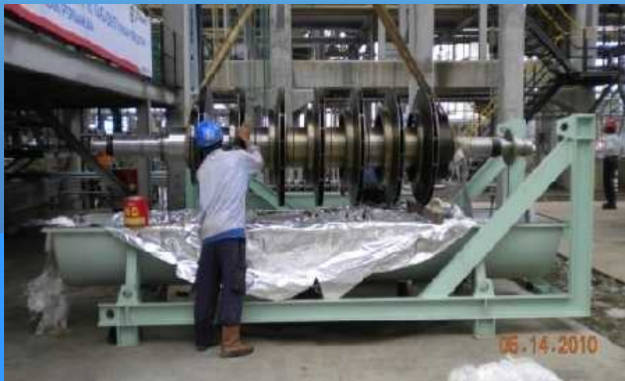
Over Haul for Turbine Compressor
