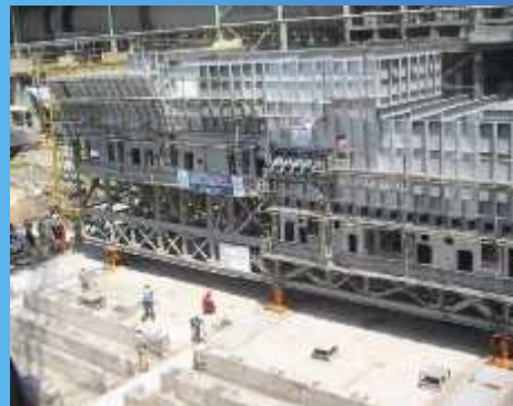
Assembly and Shifting Grate Cooler
