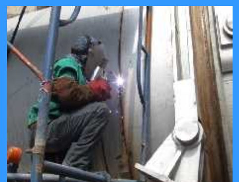
Welding Shell Kiln
