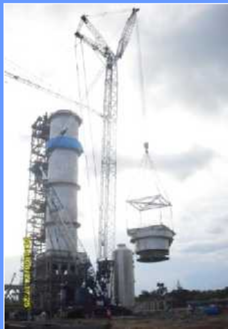
Installation for Prilling Tower
