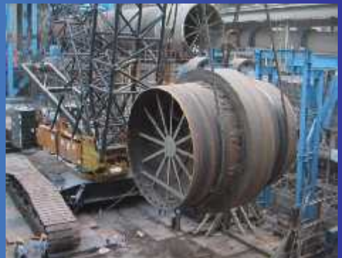
Installation for Kiln & Tire
