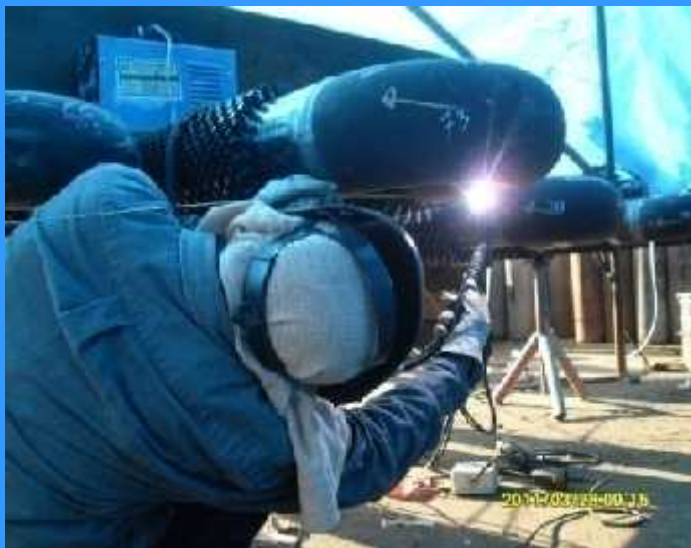
U - Bend Tube Welding
