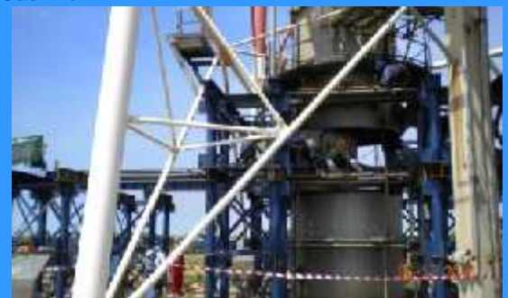
Replacement for Flare Shell Gas Drum
