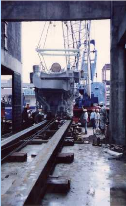
Installation for Engine Generator
