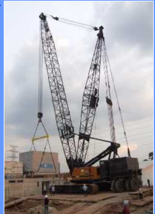
Installation for Turbine Generator
