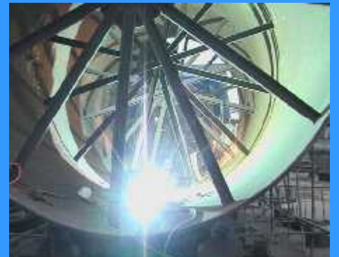
Welding Shell Kiln
